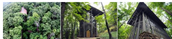
Figure 6. Photographs of Thorncrown Chapel.
