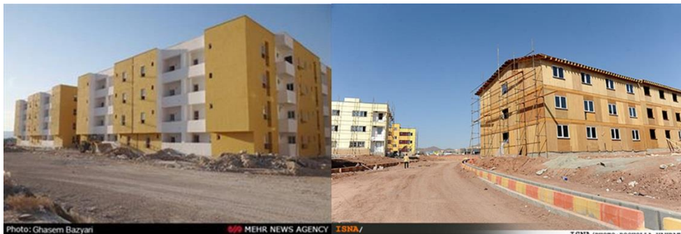
Figure1. © Mehr Housing project, Parand, Tehran 13
