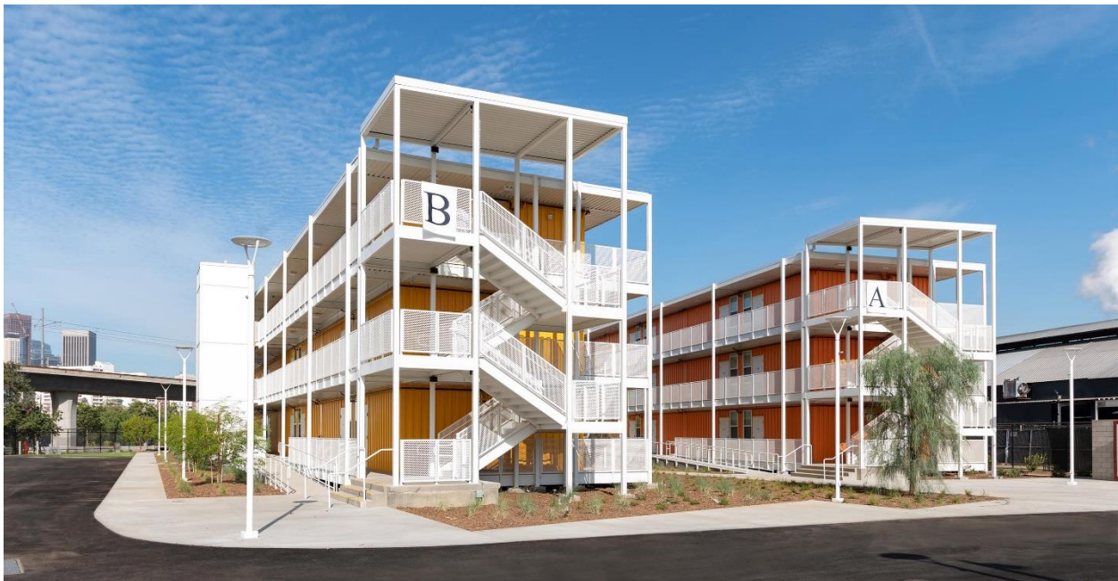
Figure 4.2.1 Rendering of shipping container buildings that make up the Hilda L. Solis Care First Village
