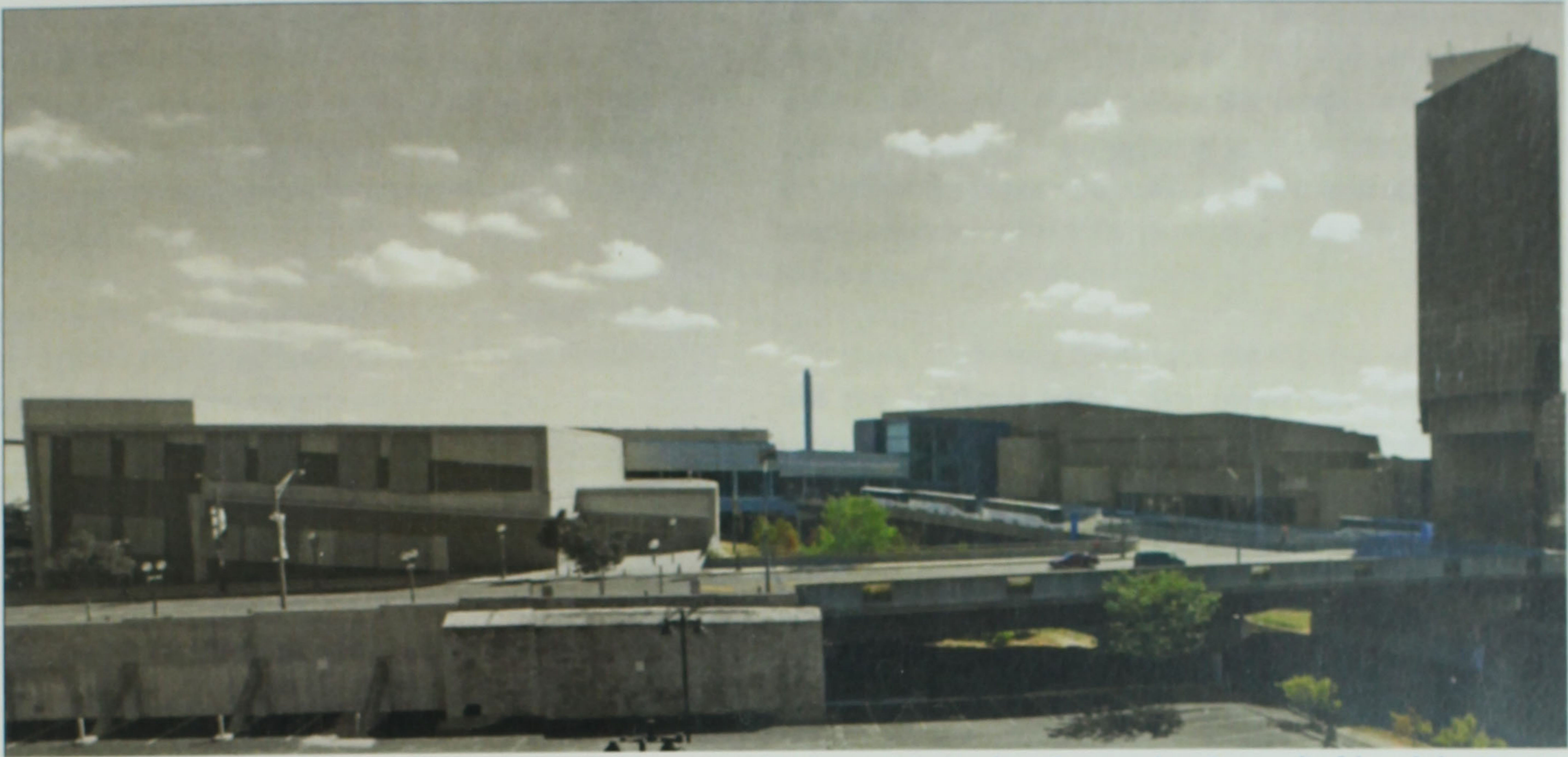
Figure 3 The new station as proposed is located between the Greater Columbus Convention Center (Left) and the Hyatt Regency (Right)
