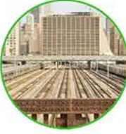
Abandoned railway makes the texture looks even more dilapidated
