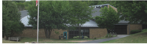
VIEW FROM SOUTHWEST
