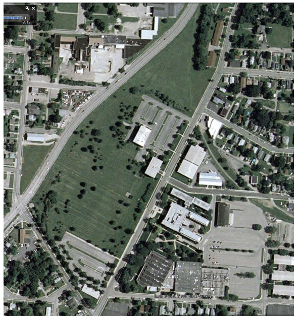
2004, AK Steel Corporate Headquarters
