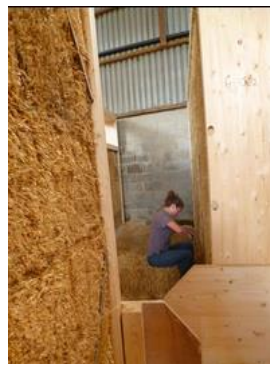
Figure 8. House Built by ModCell
