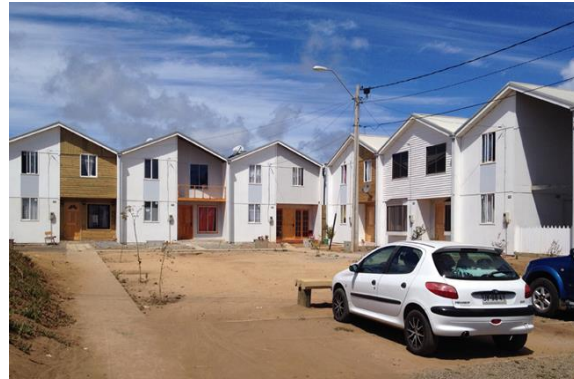
Figure 16 - Villa Verde Housing complex in Chile. The core or incremental housing model allows for owners to safely expand as their needs and budget allow (Photos by Elemental)
