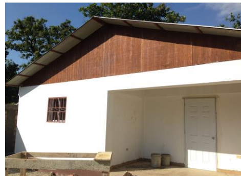
Figure 20 - E2E's model house under construction in Leogane, Haiti (Photo by author)
