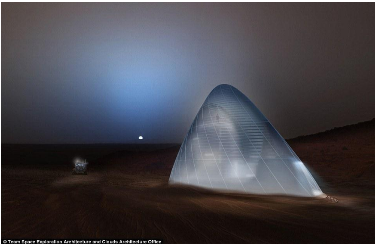
(Fig:1) Mars Ice House is 3D printed from translucent ice, which shields the crew from radiation and transforms into a glowing beacon in the Martian night.
