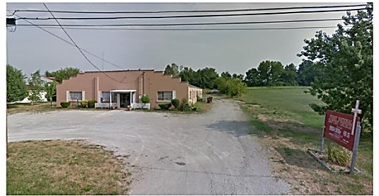
FIRST BAPIST CHURCH, FORTWAYNE, INDIANA Source: Google Earth Street View Image
