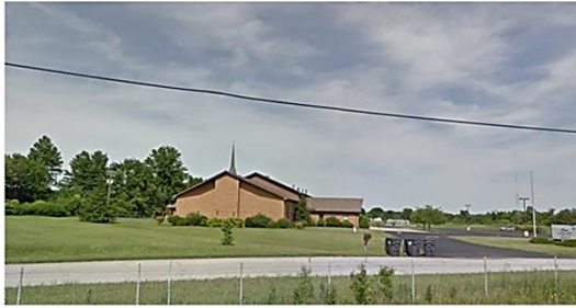
PROPOSED MOSQUE (LIQUID CHURCH), FORTWAYNE, INDIANA Source: Google Earth Street View Image
