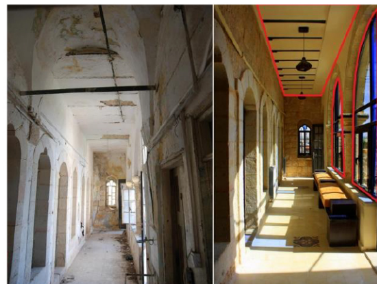
Fig. 3: Birzeit Municipality Guest House before (left) and after (right)
