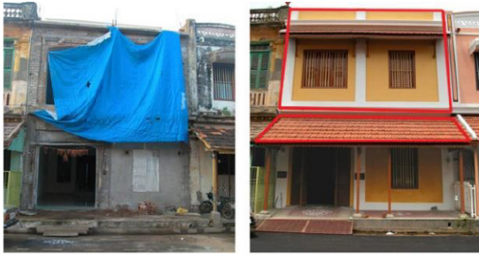
Fig 6: before (left) and after (right) restoration
