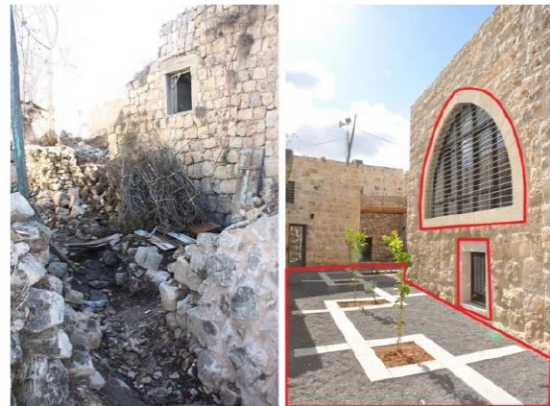
Fig. 1: upgrading the building environment
