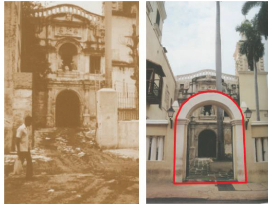
Fig 4: Convent of Belen before (left) and after (right) restoration
