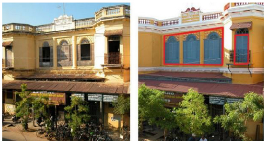
Fig 7: before (left) and after (right) restoration
