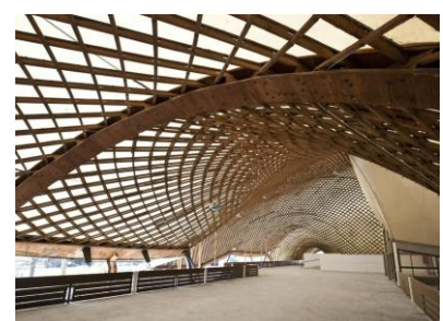
Views of 4 layered grid shell with bracing and Grid shell supports with concrete and posts.
