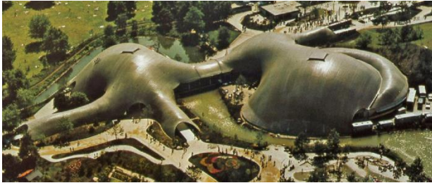
From flat to curved: the forces along the boundary cause the wooden laths to bend into a curved shape
