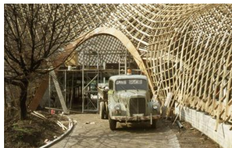
Views of 4 layered grid shell with bracing and Grid shell supports with concrete and posts.
