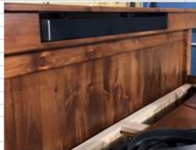
Speaker Bar Installed
