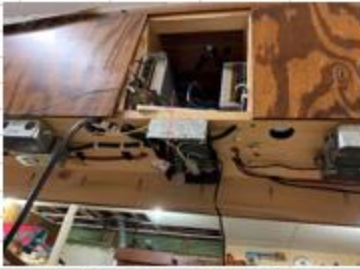
Beginning of wiring of sub-headboard outlets
