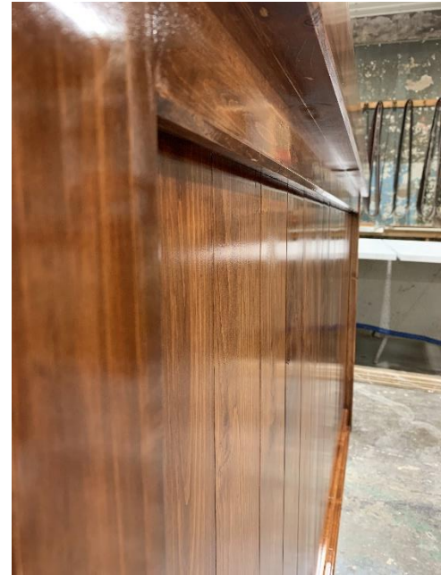
Figure 19: Wood Finish on Footboard
