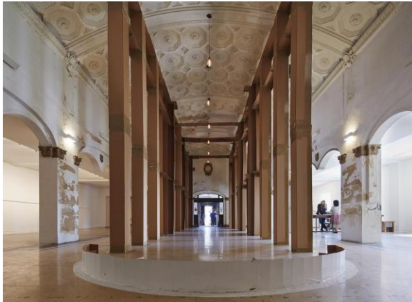
Stony Island Bank before and after renovation photo from google
