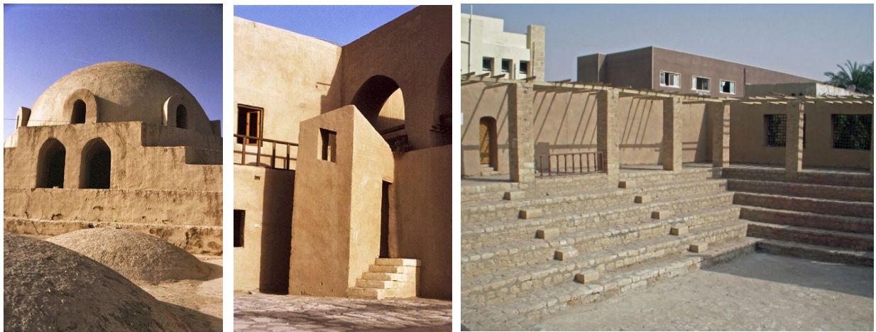
Fig 34 : Different view of New Gourn Village ; Photo : Google.
