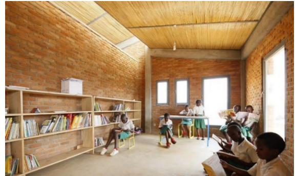
Fig 21: View of the library, a papyrus-reed dropped ceiling provides natural ventilation and diffused light; Photo: Iwan Baan.
