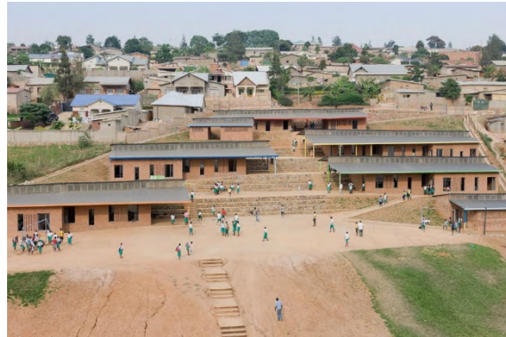
Fig 17: View of the buildings on the sloped site; Photo: Iwan Baan.
