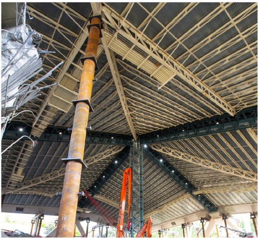
STEEL STRUCTURE: CONCRETE ROOF SITS ON ROOF JOISTS AND FOUR ORIGINAL TRIANGULAR SECTION CONNECTED TO LARGE CONCRETE ABUTMENTS
