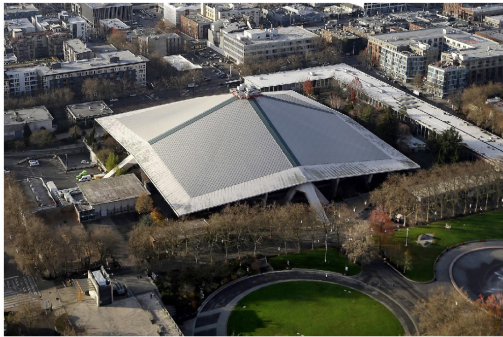
ROOF STRUCTURE: CONCRETE ROOF ON METAL PANELS WITH STANDING SEAM ALUMINUM PANELS ON EXTERIOR
