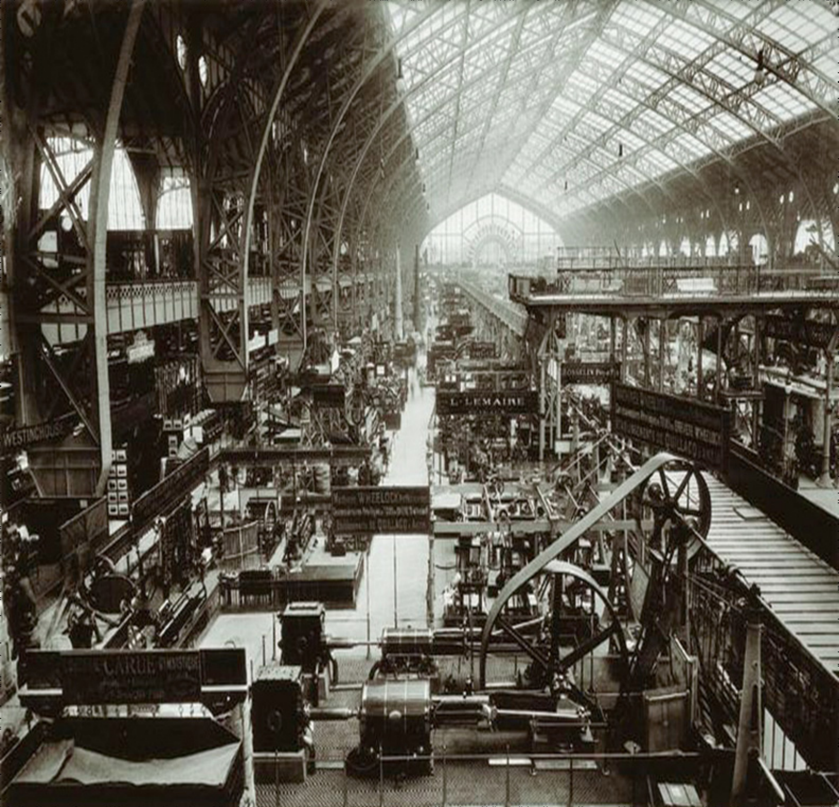
Figure 07: Hall of Machines, Paris Expo 1889
